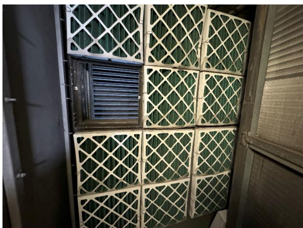
New panel filter frame and filters
