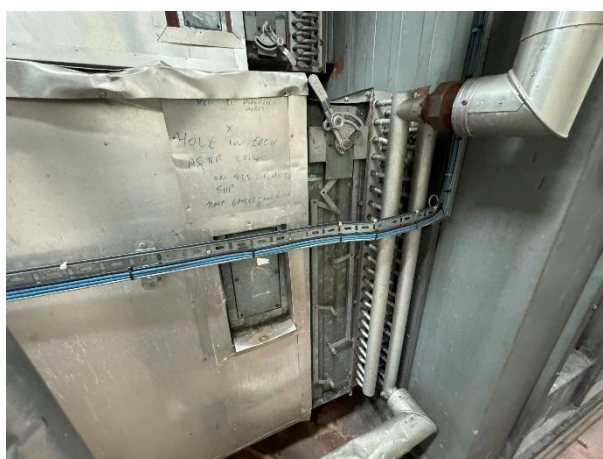
Duct mounted coil, VCD, and obstructing cabling
