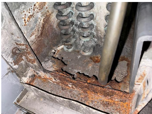
Corrosion on CHW coil headers
