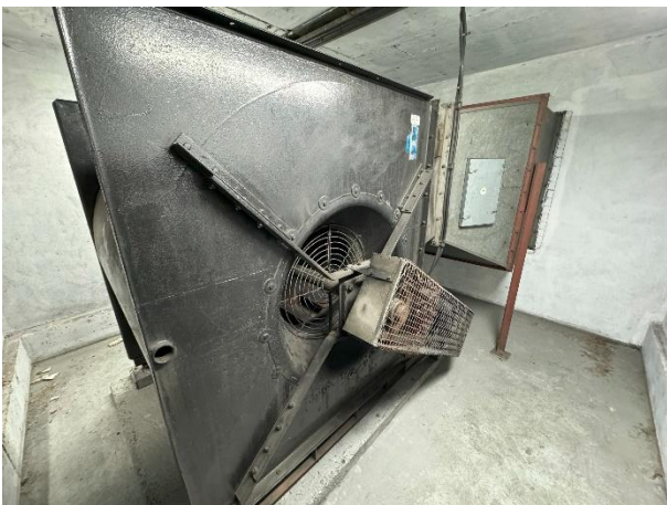
Belt driven fan and attenuator
