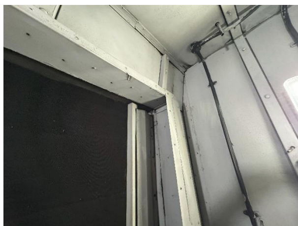
CHW cooling coil buckled casework
