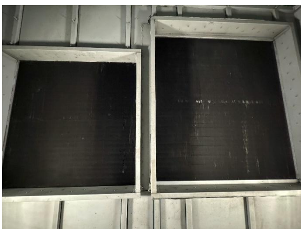
Duct mounted coils
