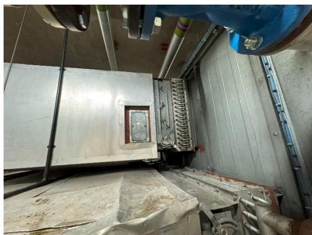
Duct mounted coil and VCD
