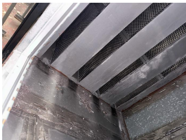
Duct mounted attenuator
