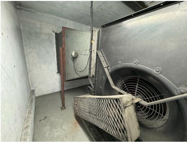
Belt driven fan and attenuator
