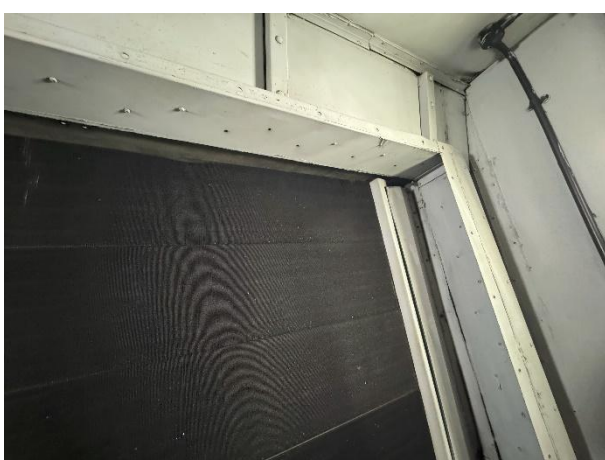
CHW cooling coil buckled casework
