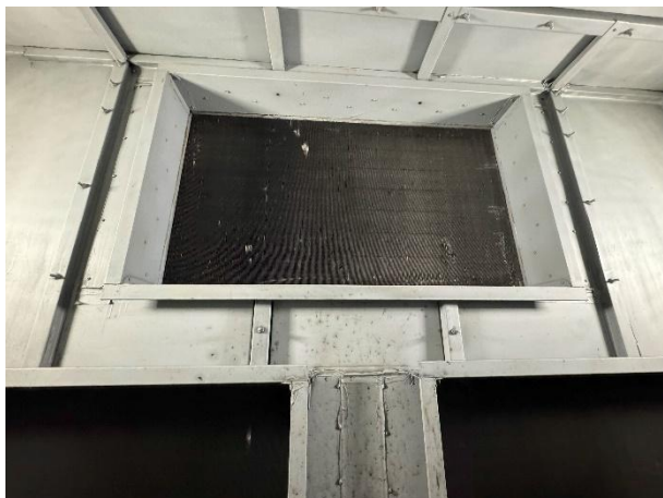
Duct mounted coil
