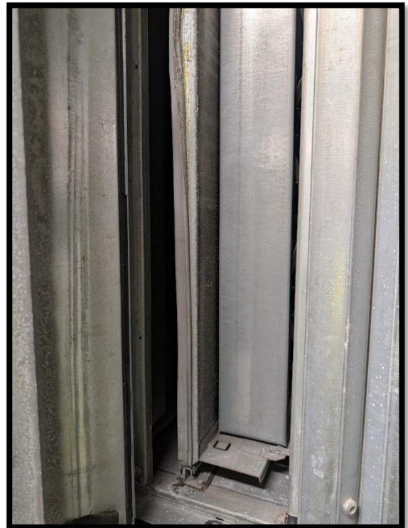
Supply panel filter section
