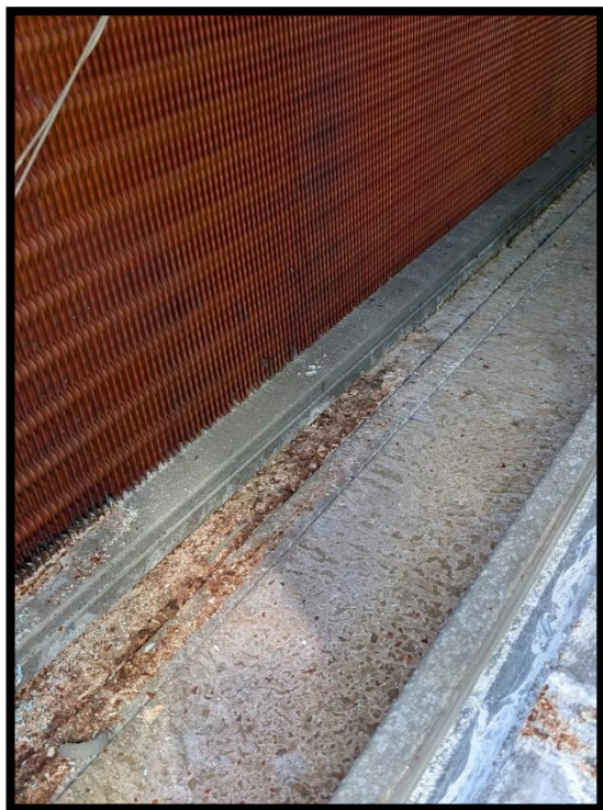
Heating Coil Corrosion
