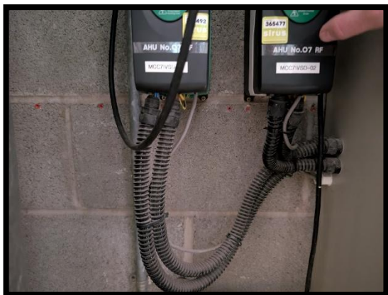
Invertors Manually Set to Reduced Duty
