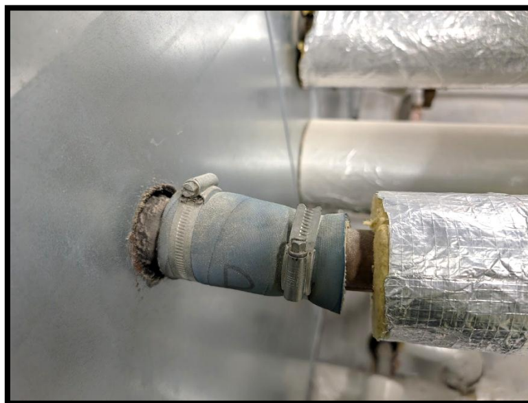
Missing Flange - Air Leak
