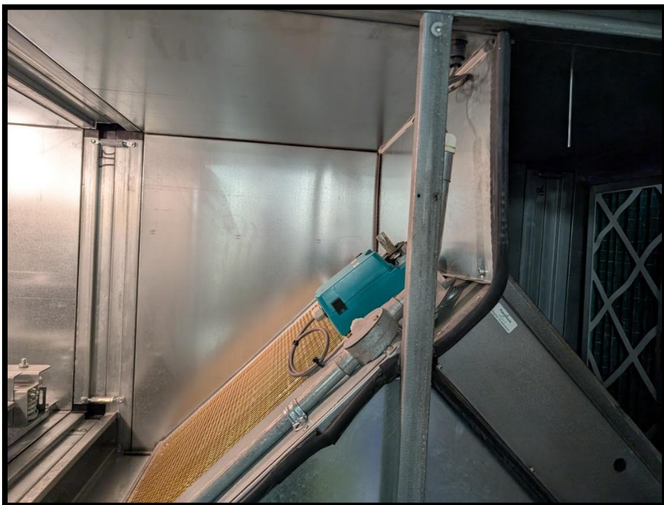
Exhaust heat exchanger section
