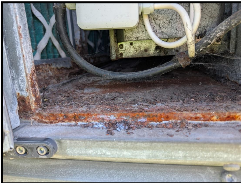
Intake Debris/Corrosion
