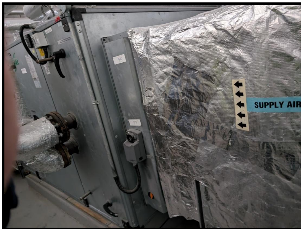
Inaccessible Damper/Intake Section
