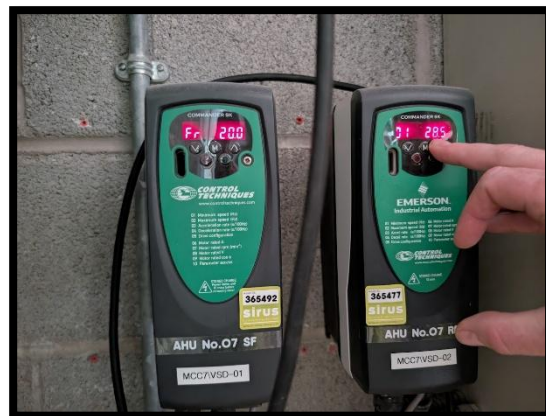
Invertors Manually Set to Reduced Duty
