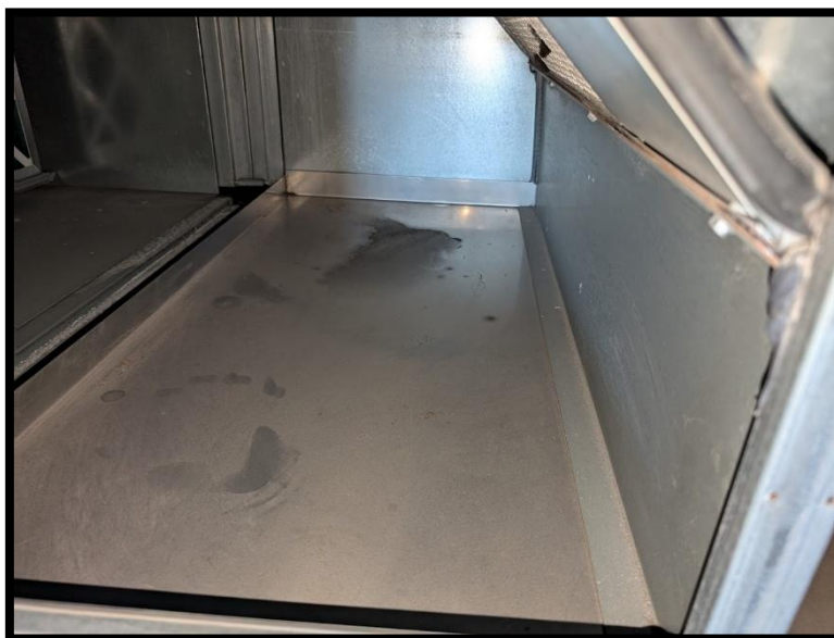
Debris Build Up Air Off Side Heat Exchanger
