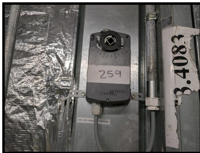
Exhaust Damper Actuator
