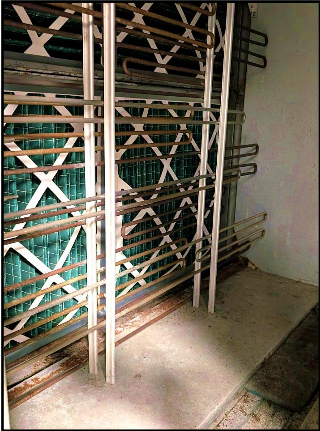
Electric Heater Battery Corroded and Located 150mm From Panel Filters.
