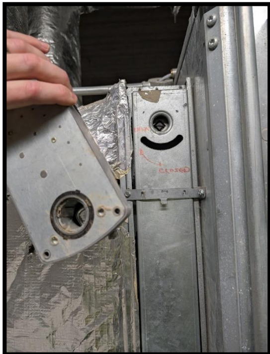
Missing Actuator on Intake Dampers
