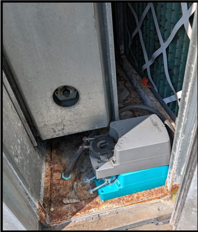
Discharge Section Corroded. Damper Spindle Snapped
