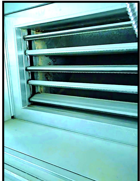
Air Off Damper Side – unable to access air on, signs of debris/corrosion through dampers
