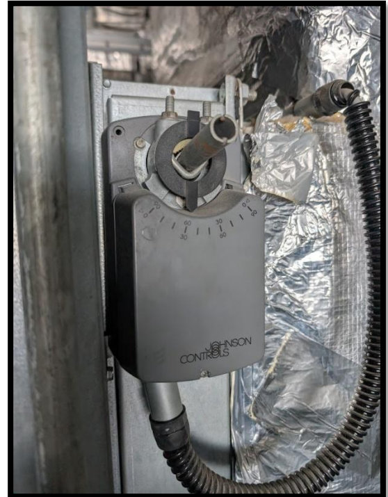
Supply Damper Actuator
