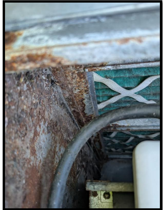
Intake Section Corrosion
