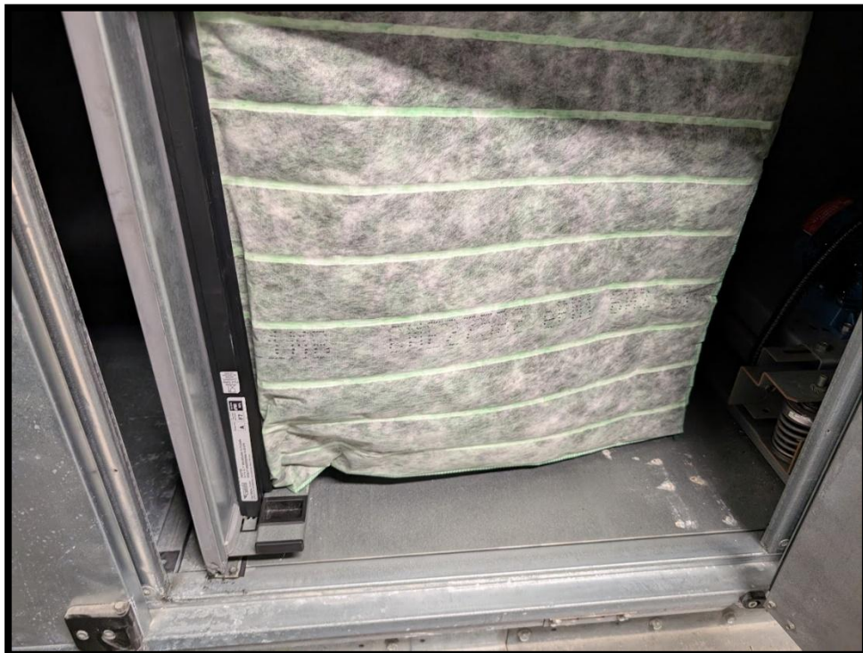
Supply Fan Section Bag Filters
