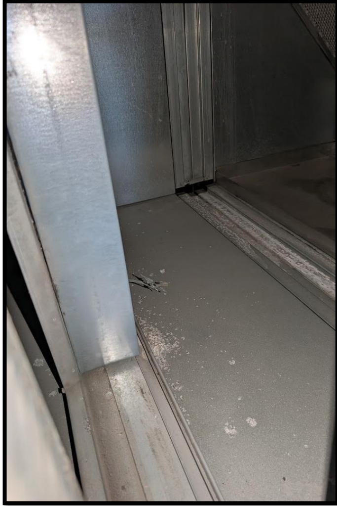
Intake Filter Section debris/Corrosion
