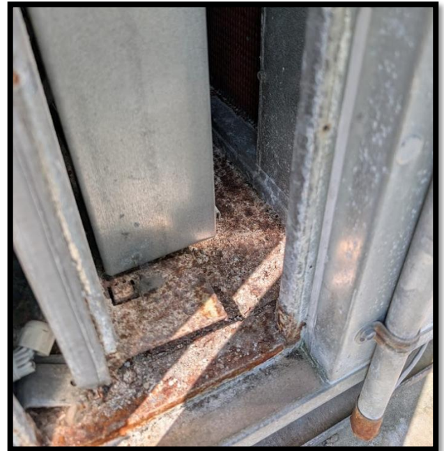
Intake Section Corroded
