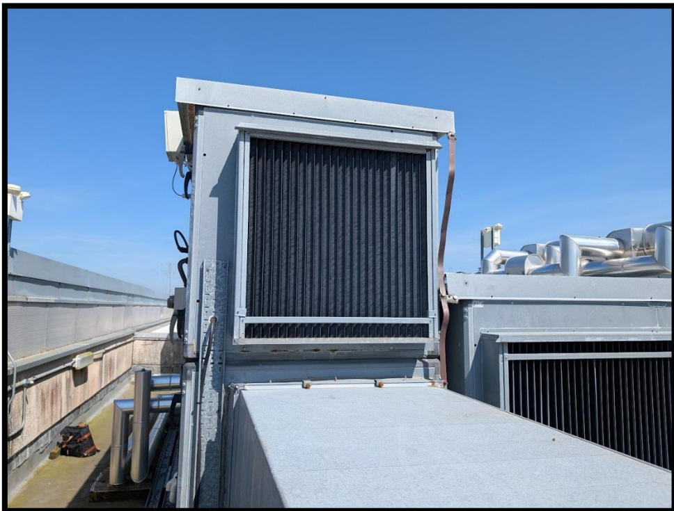
Not Fit For Purpose Intake
