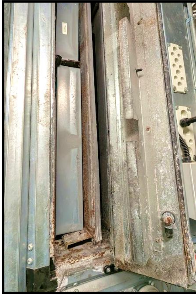
Intake Filter Section Collapse/Corrosion
