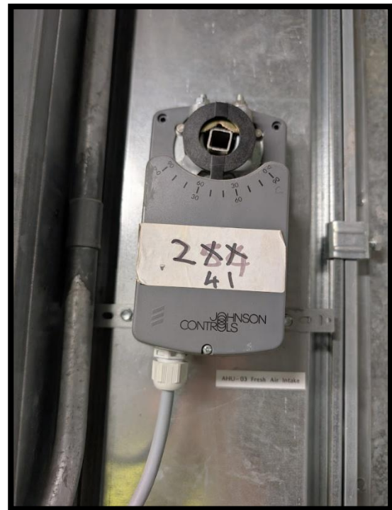
Supply Damper Actuator
