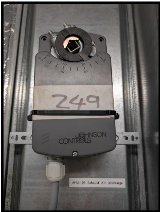
Exhaust Damper Actuator
