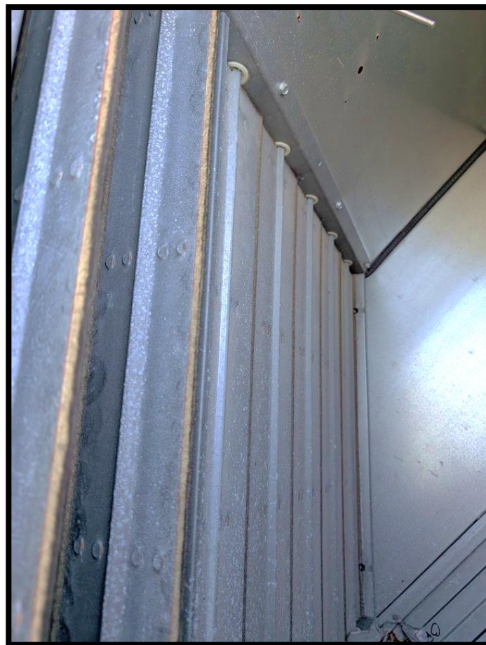
Microbial Growth on Heat Exchanger
