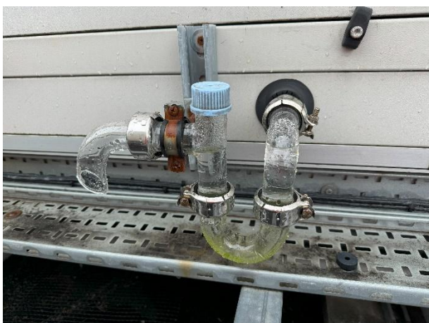
Glass trap for plate heat exchanger
