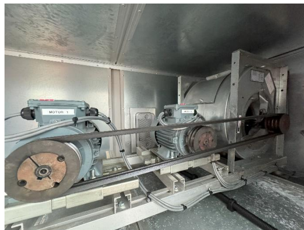
Belt driven extract fan with run and standby motors
