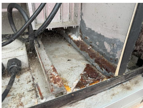
Corrosion in fresh air intake section
