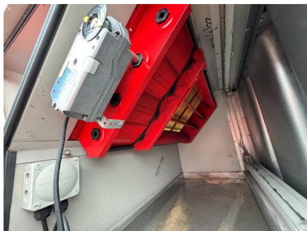
Air off side of plate heat exchanger in extract air stream face and bypass damper
