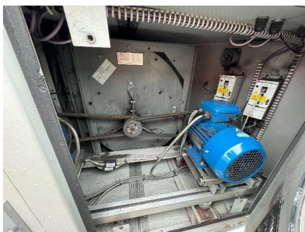
Belt driven SISW supply fan with run and standby motors
