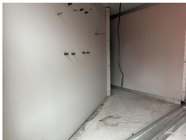
Divider within fan section to separate motors from air stream
