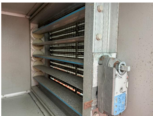
Fresh air inlet damper and actuator
