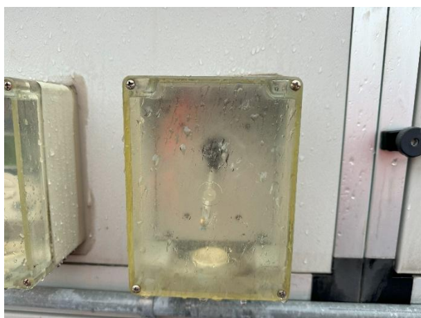
Missing inverter keypad
