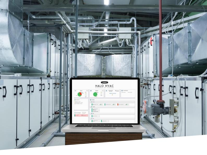
loT can facilitate predictive maintenance by collecting and analyzing data from HVAC equipment. Sensors can detect early signs of potential issues or equipment failures, allowing for proactive maintenance to prevent breakdowns and reduce downtime.
