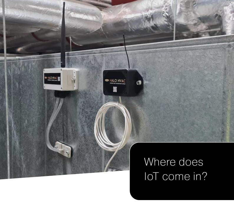
HALO HVAC IoT sensors enables real-time monitoring for quick issue resolution, energy efficiency optimization, predictive maintenance, and remote control.
